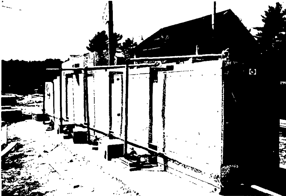
Fig. 24 View of Ammonia Stripping Unit
